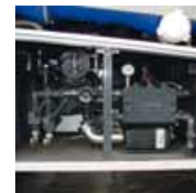
High-pressure pump: Uraca P3-10, 127 litres per minute at 160 bar. The pump pictured is placed inside a cabinet for frost protection.
